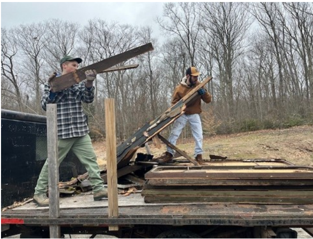
We filled 2 dumpsters on the huge work weekend!
