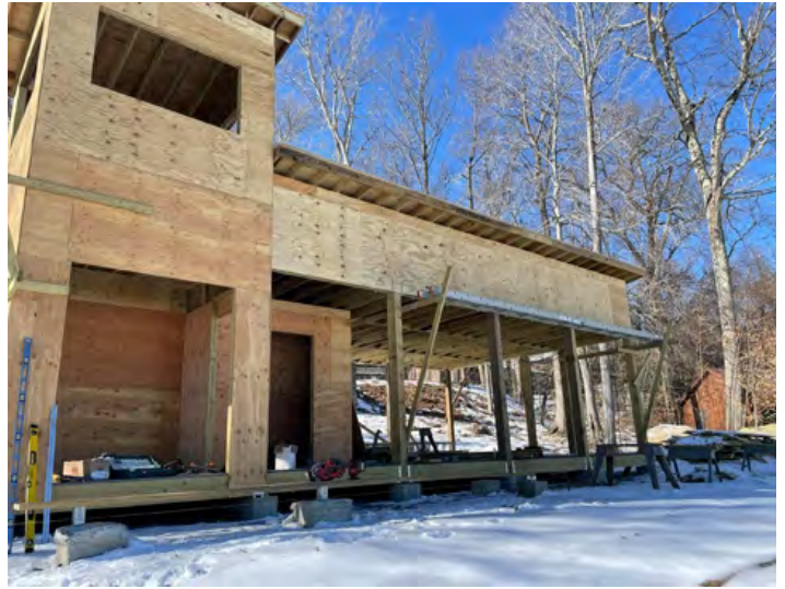
Winter work on the Pavilion.
