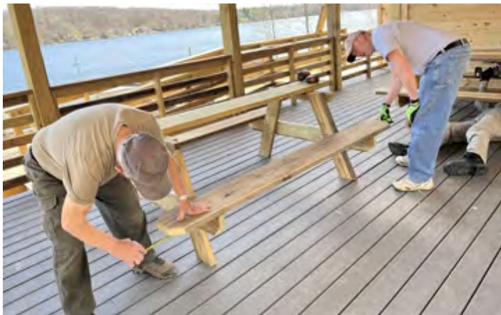
Picnic tables under construction.
