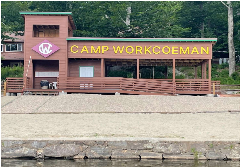
New Construction complete!
