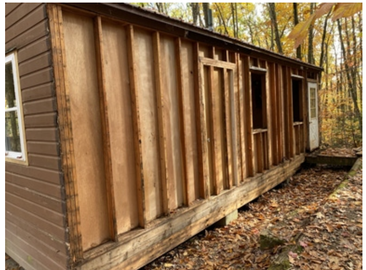
Calder rehab underway
