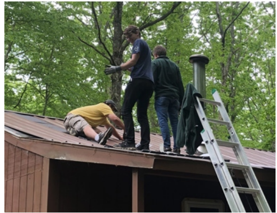
Roof work on Griffin Lodge
