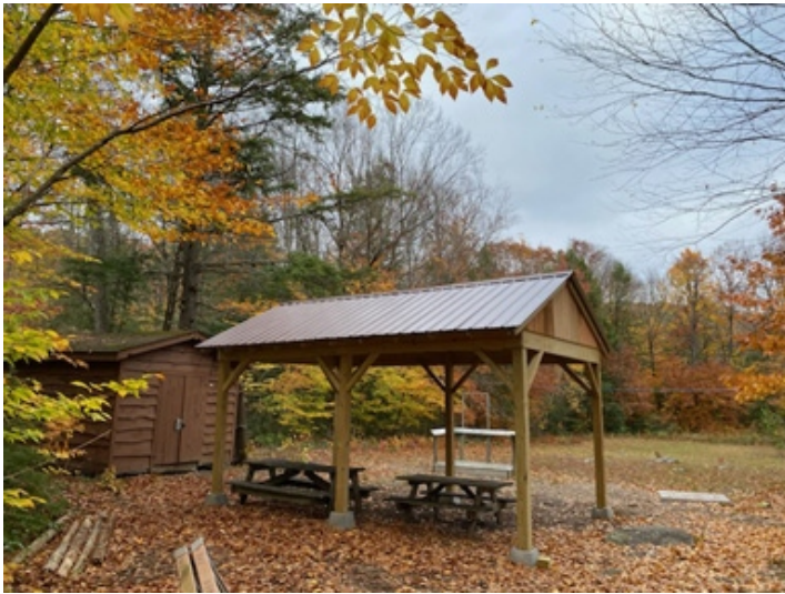
Completed pavilion at shooting range
