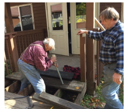
Ron DiPietro and John Klimas make repairs to porch at Dining
